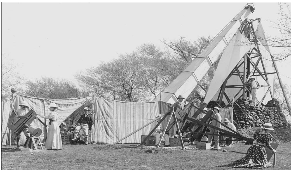
Figure 4: A scene showing the Lick Observatory party ready for the eclipse. All of the instruments are in place and the volunteers are at their practice stations. The 40-foot Schaeberle Camera with its twin wooden towers dominates the scene.
